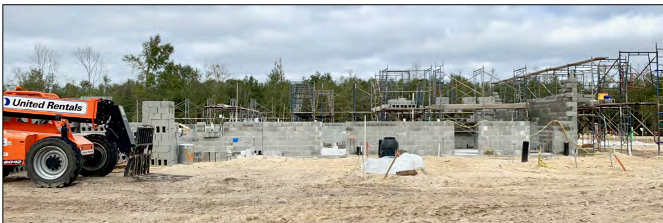
The Mother House under construction.
