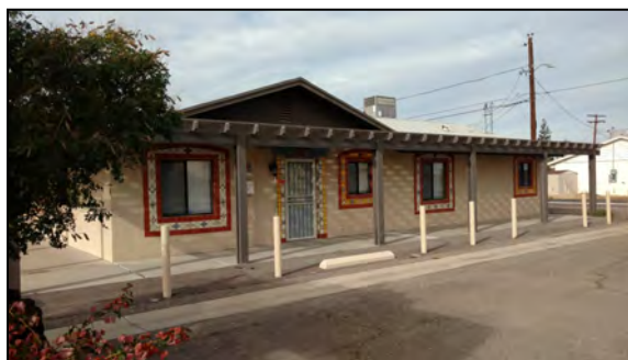
The new church in the Phoenix area.
